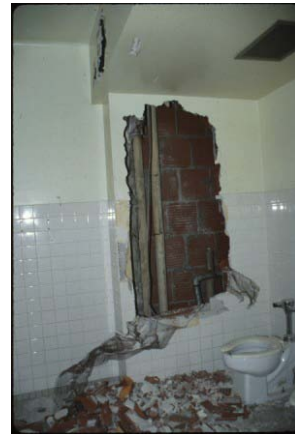
Plaster on speed tile
