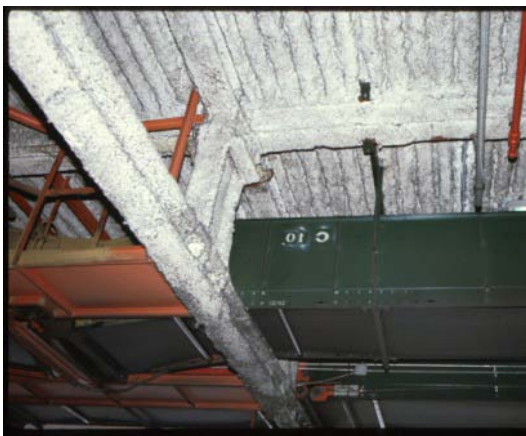
Fibrous sprayed fireproofing
