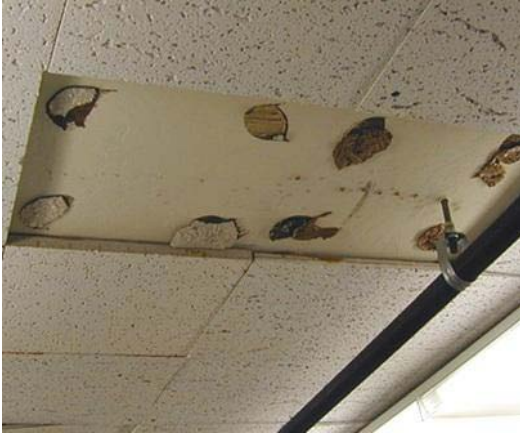
Glued on (laminated) ceiling tiles
