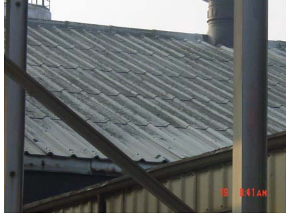
Corrugated Transite Siding/Roofing
