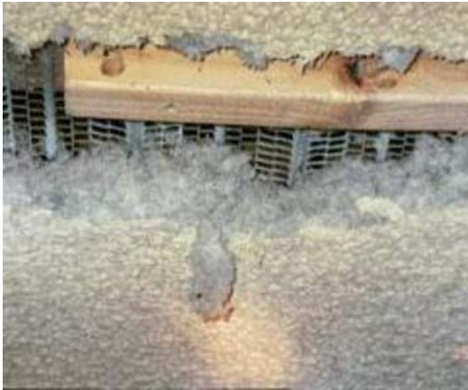
Sprayed limpet texture ceiling on lath
