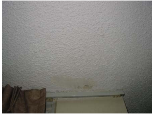
Texture coat ceiling
