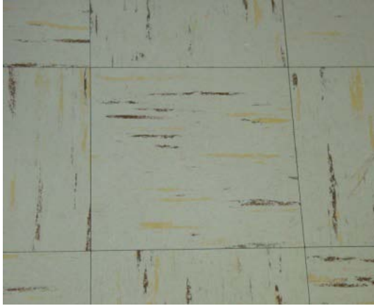
Vinyl asbestos tile
