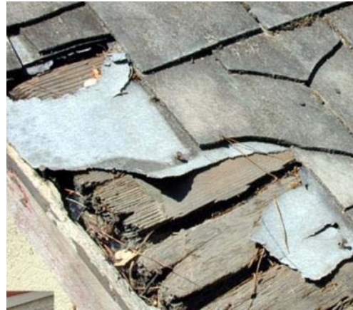
Building paper under roof tiles
