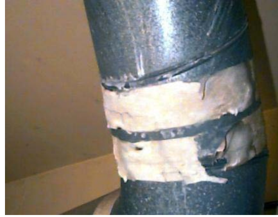
Paper on seams of duct
