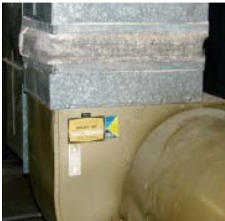
Textile Vibration Damper/Duct Connector
