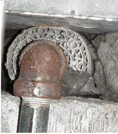
Aircell insulation (corrugated paper)
