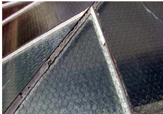
Caulking at Glazing
