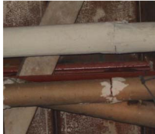
Parging cement on sweatwrap and Aircell
