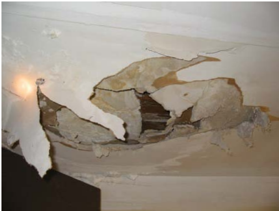
Plaster on wood lath
