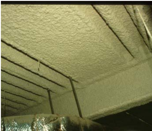
Cementitious sprayed fireproofing
