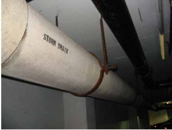
Transite Drain Pipe
