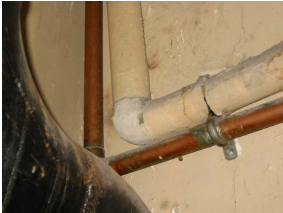
Parging cement on pipe fitting
