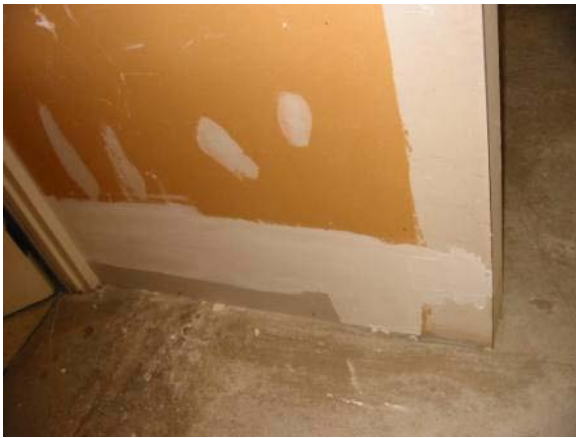
Drywall joint compound on drywall
