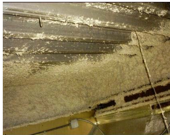
Fibrous sprayed fireproofing (beam only)
