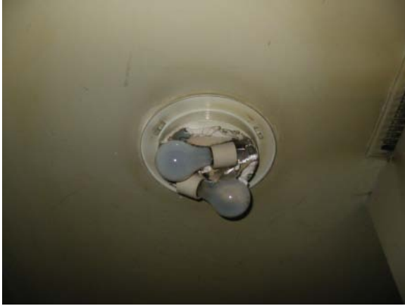
Paper heat shield on incandescent fixture
